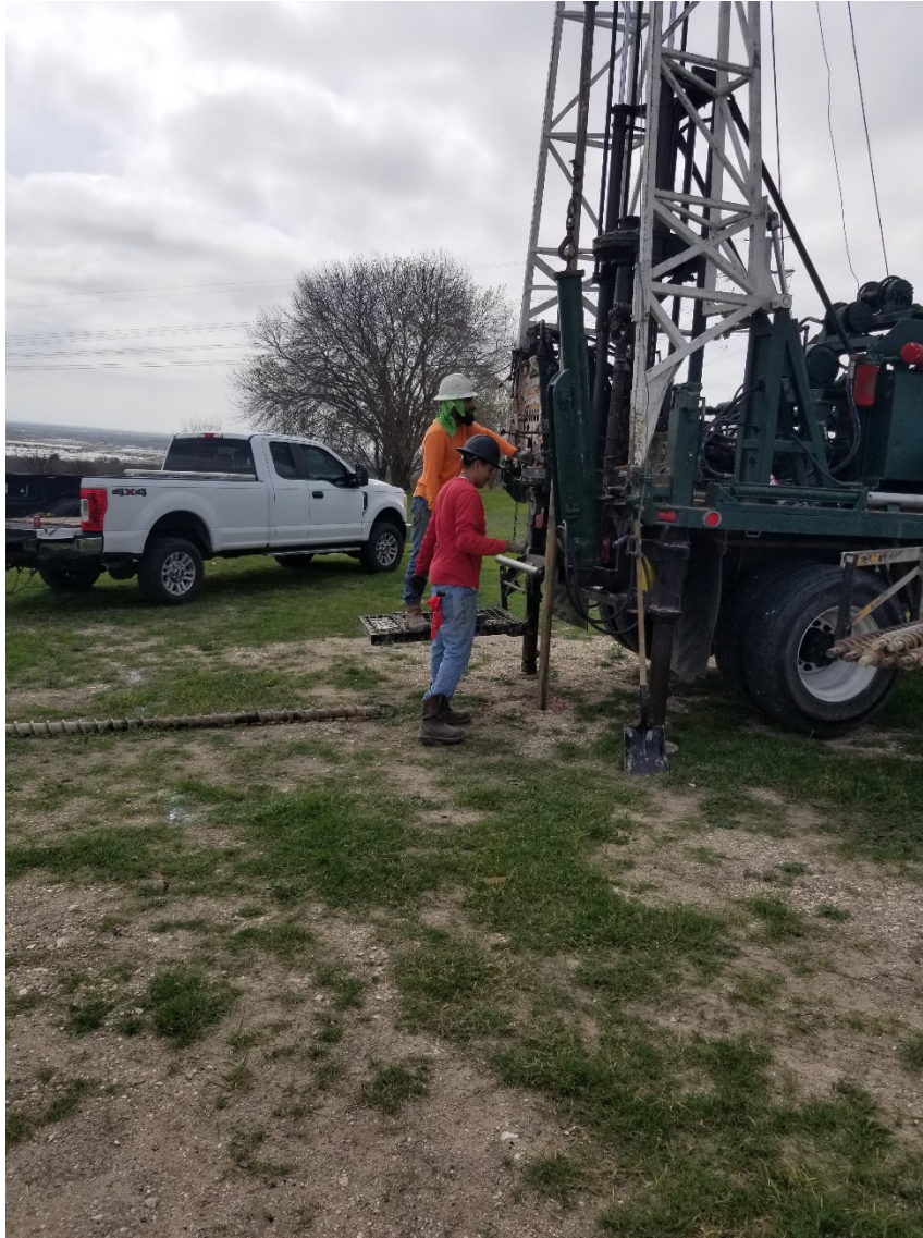
View looking at drilling operations for boring B-4.
