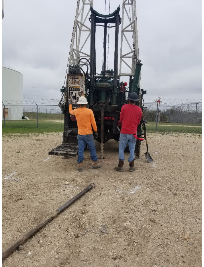
View looking at drilling operations for boring B-3.
