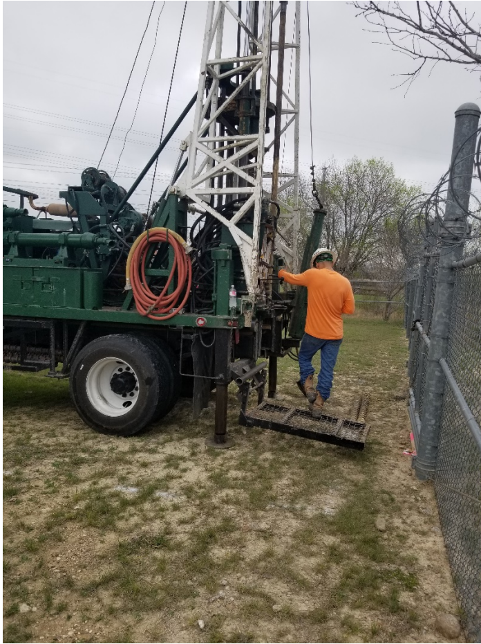
View looking at drilling operations for boring B-2.
